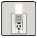
2. Plug an ordinary nightlight into the GFCI and turn it ON. The light should now be on.
